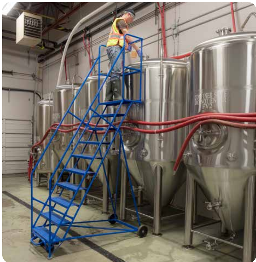
Platform ladders allow workers to perform tasks safely at the top of tanks.
