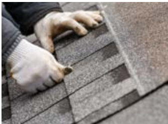
Built up roofing and felts, roof shingles/siding
