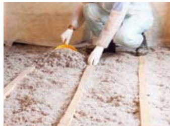
Vermiculite insulation, ceiling tiles and coatings
