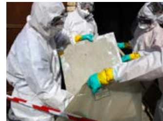
Drywall and cement sheets
