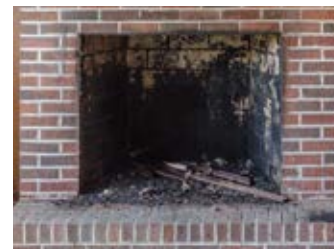
Thermal boiler and fireplace insulations
